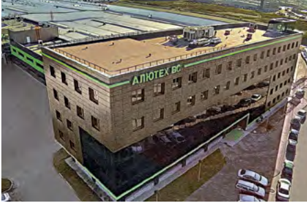
"Alutech Doors Systems" LLC
